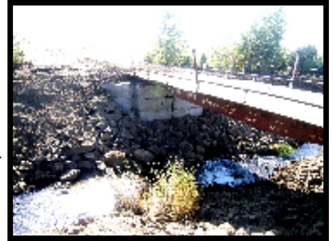
Bridge support post-construction
