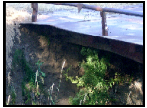
Bridge support pre-construction
